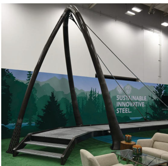
FIGURE 5 Pedestrian bridge exhibit at NASCC 2025, incorporating WAAM parts (Binder et al., 2025)
