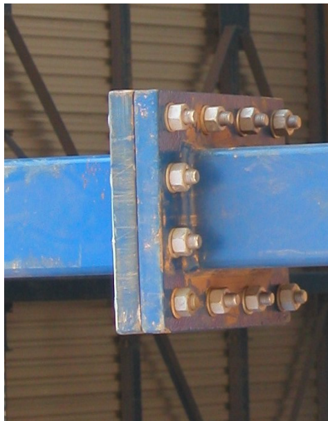
Figure 1: Four-sided bolted rectangular HSS end-plate connection in bending
