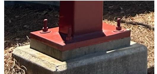
Figure 1 Rectangular HSS Column with Base Plate
