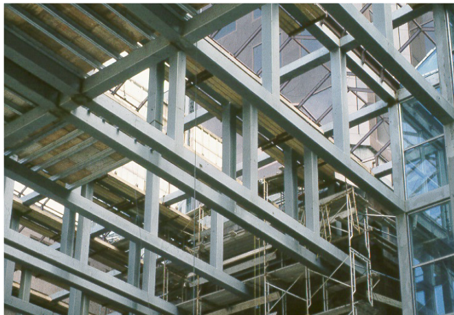
Figure 9: Square HSS-to-HSS Vierendeel Moment Connections
