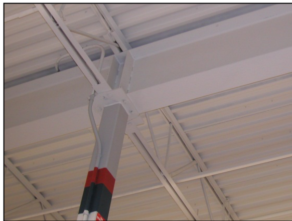
Figure 6: Continuous beam over a square HSS column
