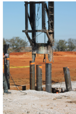
Figure 4: Pipe Piles
