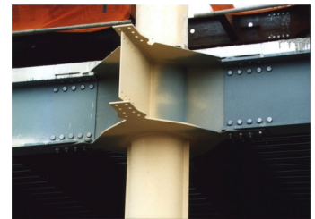
Figure 3: Moment connection to HSS column using exterior diaphragm plates
