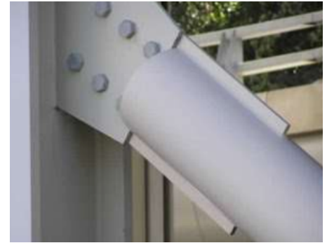
FIGURE 5 Slotted End Connection Image Credit: Atlas Tube
