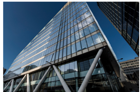
Figure 4: Concrete-Filled HSS at London's Moorgate Exchange Photo Credit: Tata Steel and SOM/Bruce Damonte
