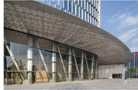
Figure 1: Concrete-Filled HSS at Ningbo Bank of China Headquarters Photo Credit: SOM/Archexist
