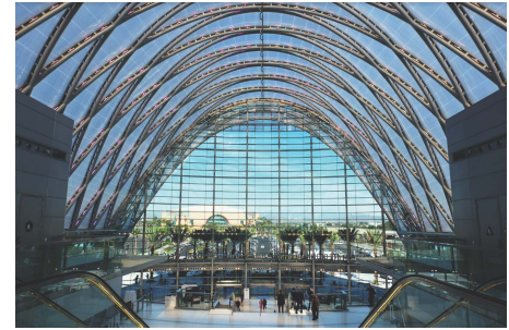
Figure 5: Anaheim Regional Transportation Intermodal Center Image courtesy of AISC/Thorton
