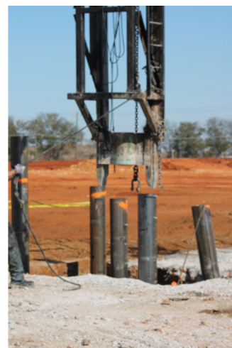
Figure 4: Pipe Piles
