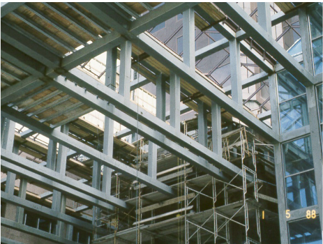
Figure 1: Vierendeel frame, using equal-width HSS members
