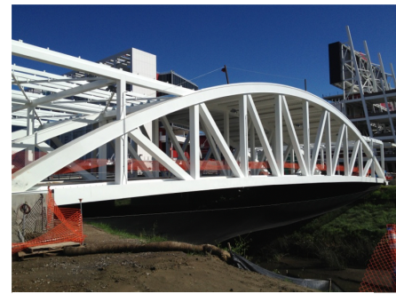
Figure 1: HSS -to-HSS Connections
