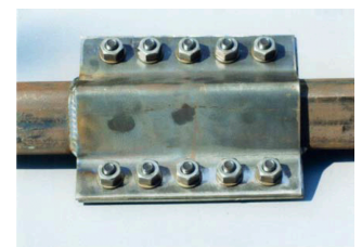
(b) after bolting together
