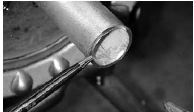
Figure 8: A minimal amount of pressure will remove the burr completely and eliminate possible flaring of the conduit end.
