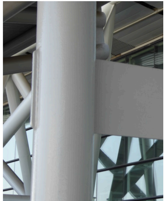
Figure 1: Example of a through plate connection to a round HSS
