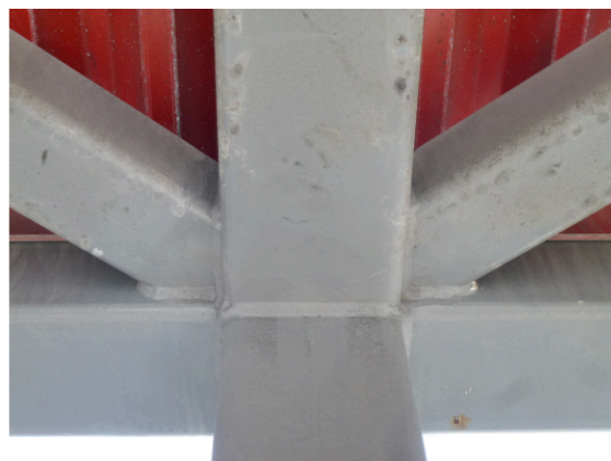
(b) Rectangular HSS KT-connection
