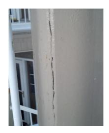
For that reason, STI recommends specifying a small weep hole at the base (or underside if a horizontal member) of the member, in addition to closing the section with cap and base plates. This small weep hole will allow any moisture that enters the section during construction or service to have a path out. If the member is galvanized, this weep hole can do double duty as a vent hole for the galvanizing process.
