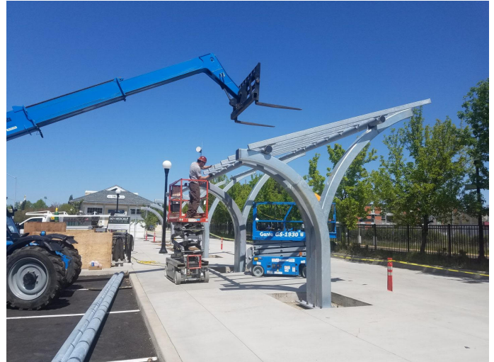
Salem, Oregon Bus Terminal Canopy © American Galvanizers Association
