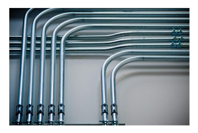
"IT'S FAR MORE COST-EFFECTIVE TO USE STEEL CONDUIT TO CARRY A BUILDING'S ELECTRICAL CONDUCTORS IN THE FIRST PLACE THAN IT IS TO HAVE TO COME BACK LATER AND INSTALL SHIELDING." Larry Maltin knows the high cost of retrofitting buildings to eliminate the effects of electromagnetic fields (EMF) on computer terminals and other sophisticated electronic equipment.
