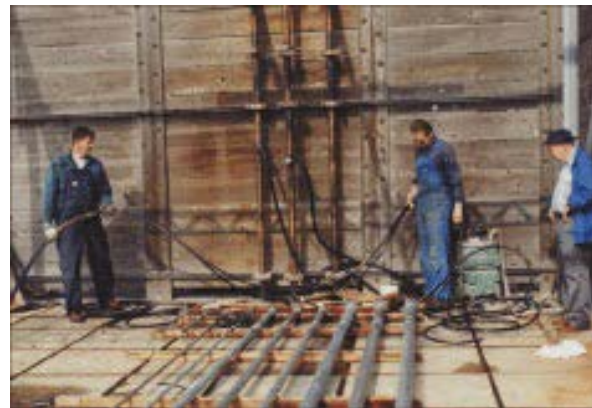
Figure 7. Electricians pulling wire, with Russ Higginbottom, Triangle Conduit & Tubing, overseeing.
