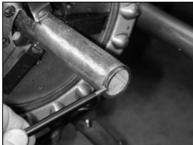
Figure 6: The roll cutter will leave a burr on the inside diameter of the conduit. The burr must be removed to ensure that the wire insulation will not be damaged during pulling.
